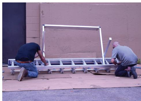
Pivot front ends of top of extreme stand into front brackets and secure with fast pins.
